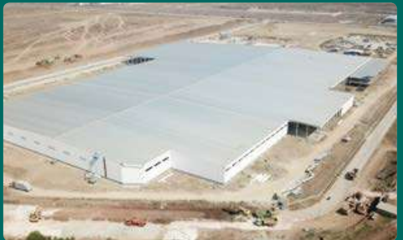
PT Kohler Manufacturing, Bekasi
